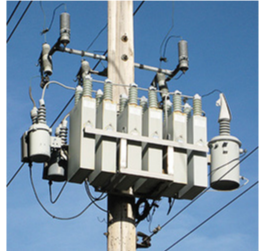
Figure 1: Pole-mounted capacitor bank
