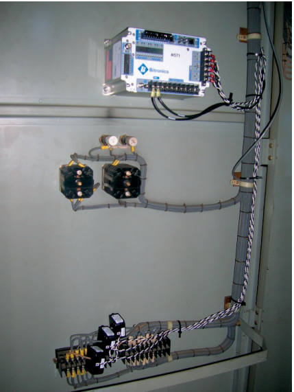
Bitronics 70 Series retrofitted on an electromechanical relay panel. Note the split core CTs on the 5A relay CT circuits.
